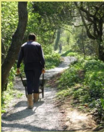
Path work at Saltburn Gill
